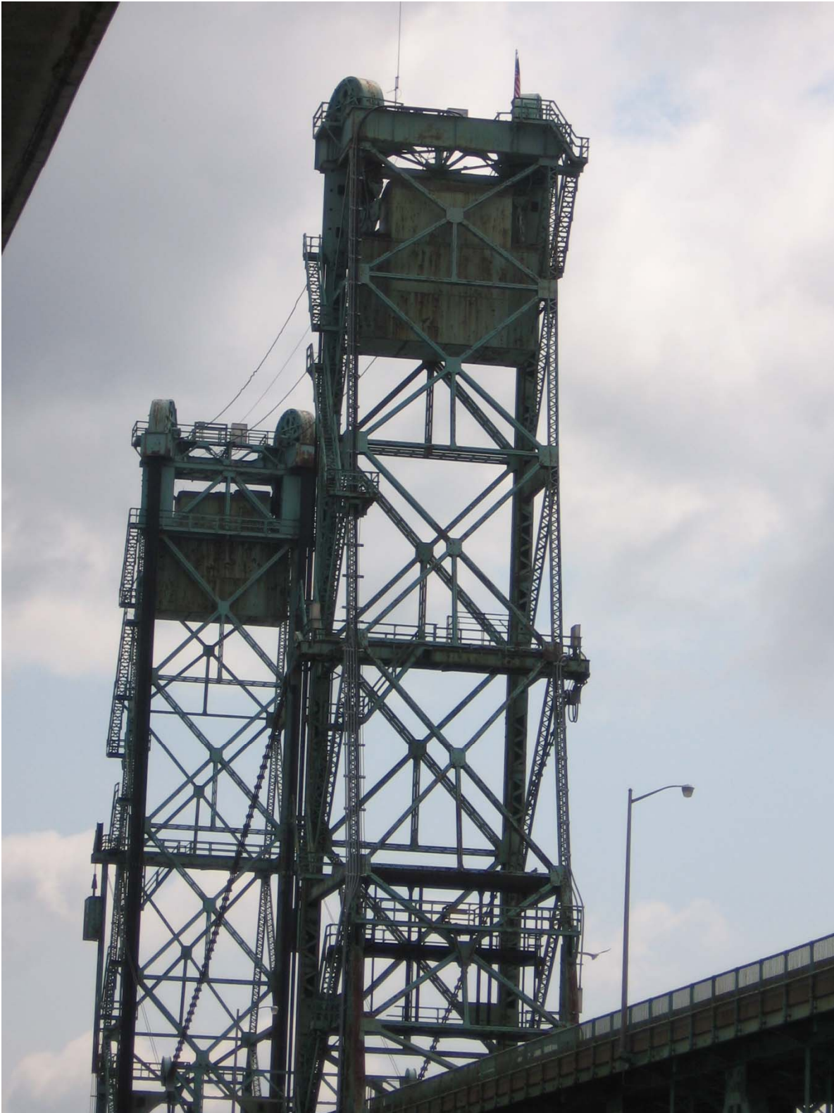
Carlton Lift Bridge
